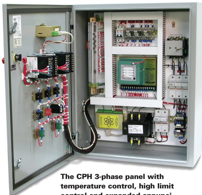
**The CPH 3-phase panel with temperature control, high limit control and expanded annunciation.**
